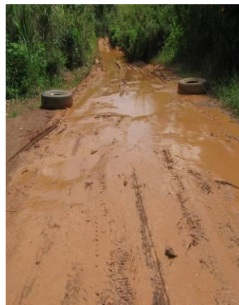
Path degraded by trucks
