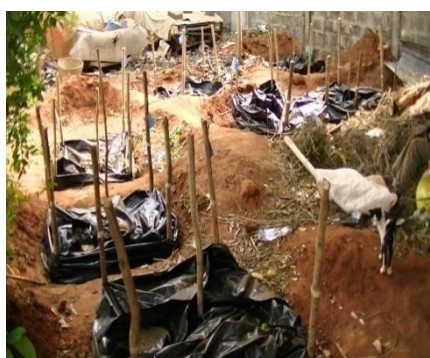
Photo 1h: Partial view of the closed pits
