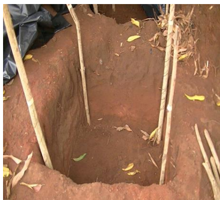
Photo 1 a: 0.5m 3 pit delimited by four rods
