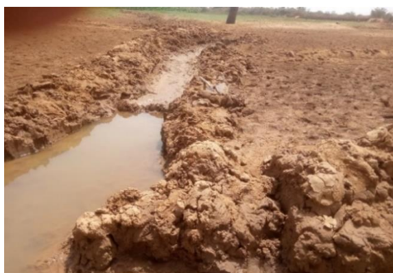
Photo 3. Opening trenches in the reservoir basin of a dam
