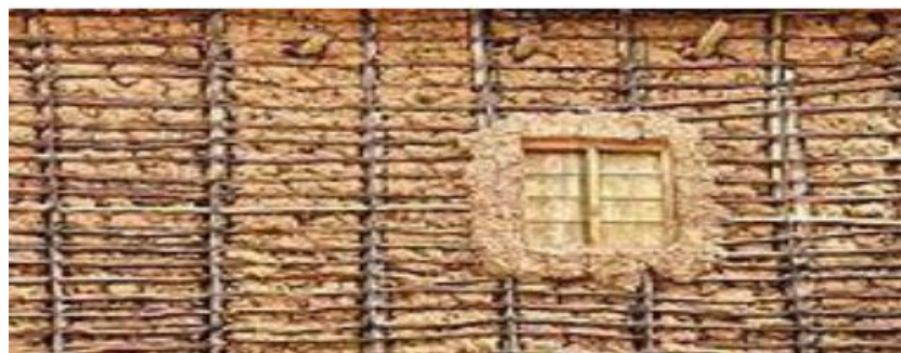
Fig. 2. Construction Torchis
