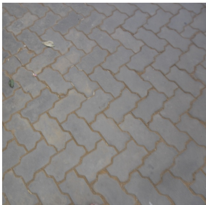
Fig. 4. Paver Blocks for the Drainage of Water
