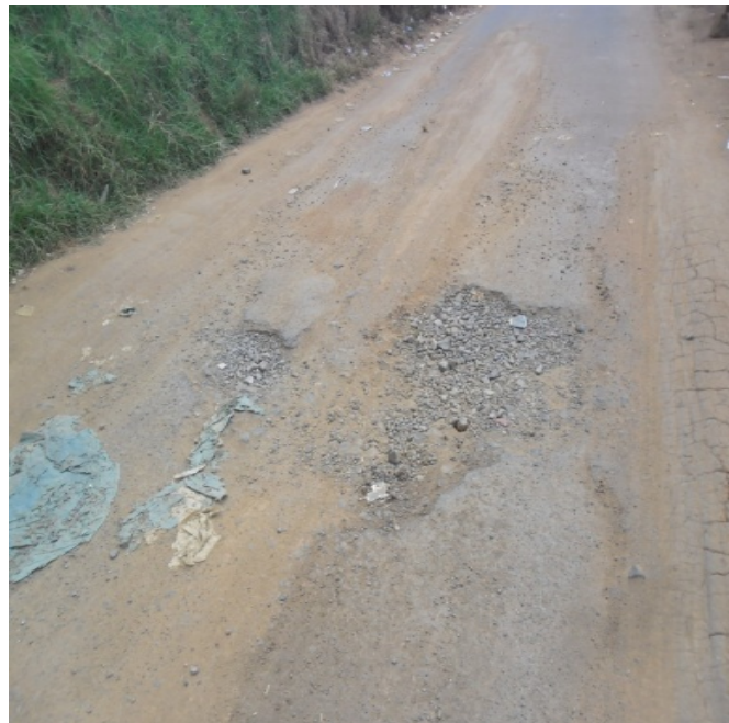
Fig. 1. Formation of Ruts at Pillicombai
