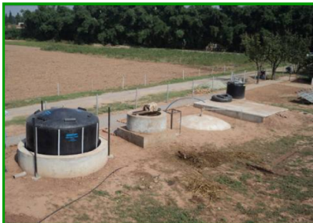
Fig. 1 Two different type of Biogas Digesters Installed at NARC, Pakistan
