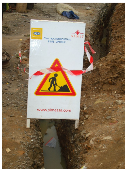
Figure 4: The building of an optical fibre network
