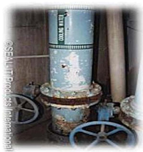
**Fig. 3. Crevice Corrosion in a Flange**
