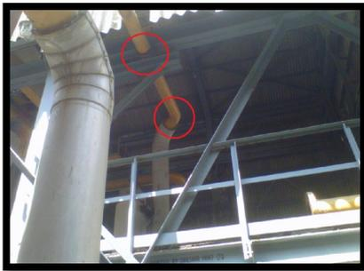
Fig 4: Points of heavy vibration (on-site location)
