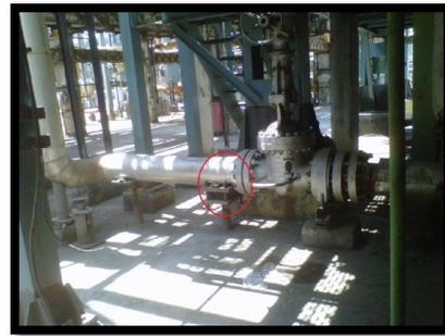
Fig 5: Points of heavy vibration (on-site location)
