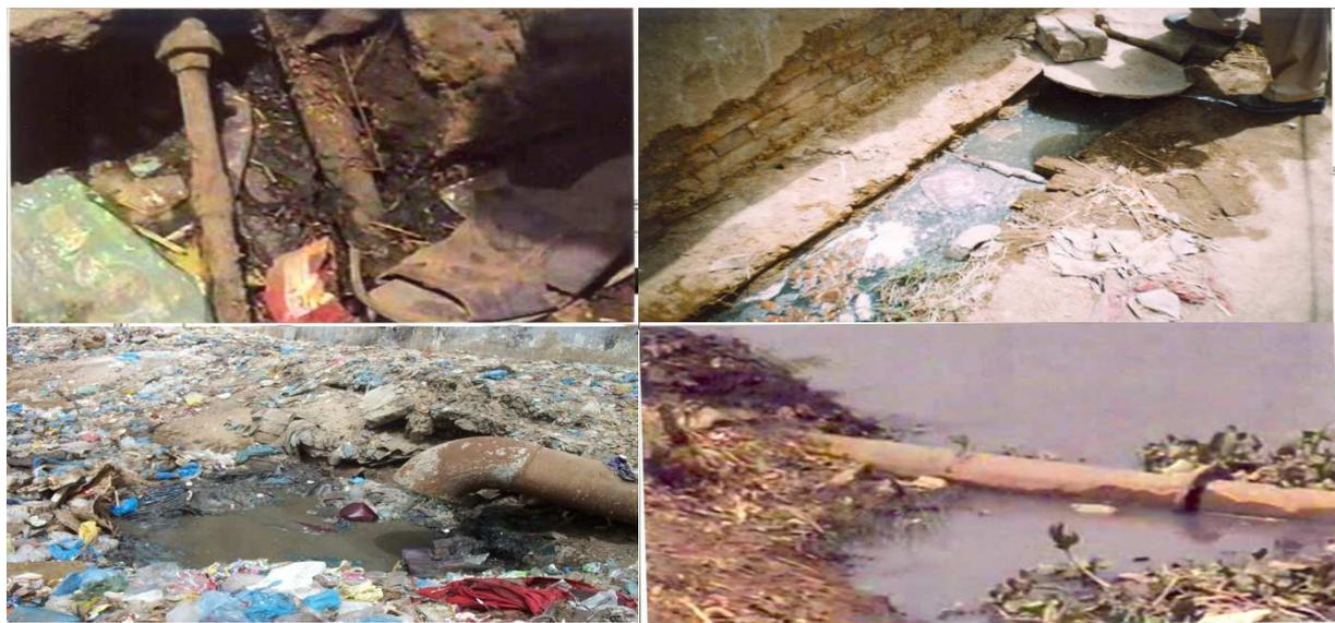
*Figure.3. Drinking Water Pipes Passing Through Manholes/Drains*
