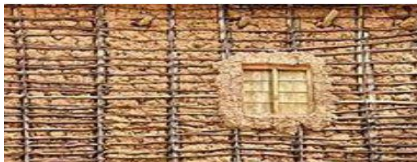
Fig. 2. Construction Torchis
