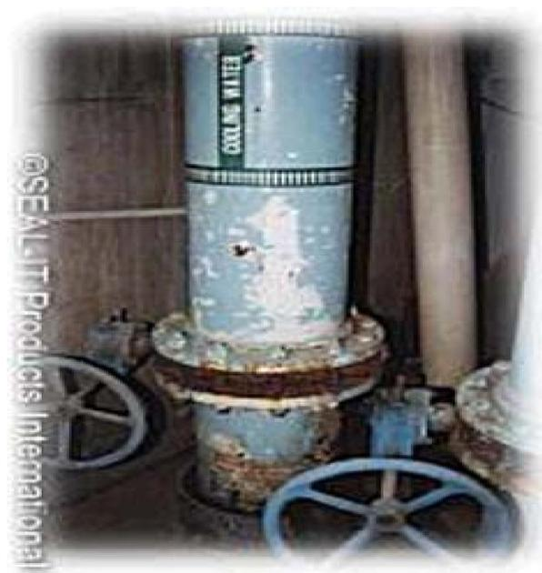
**Fig. 3. Crevice Corrosion in a Flange**
