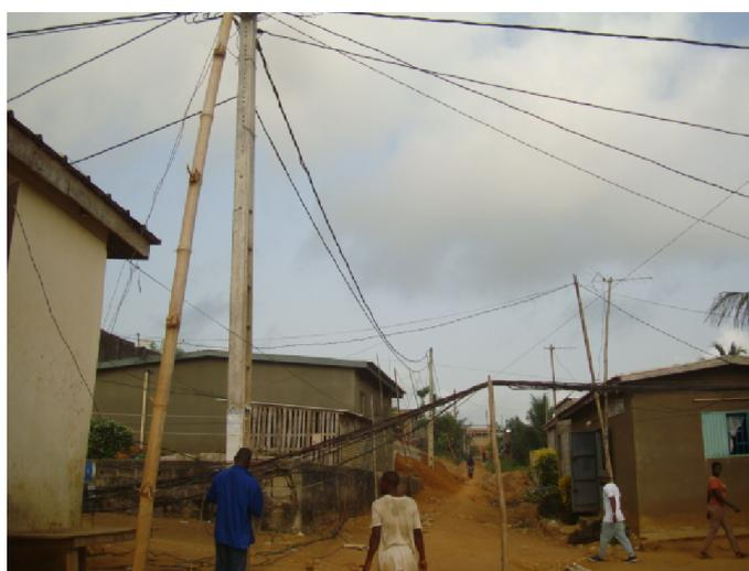
*Figure 3: anarchic connections of electric cables*
