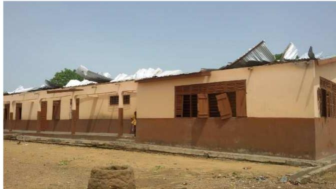
**Figure 1: Damages to a school building by the 10/05/2016 rainstorm in Bongo**
