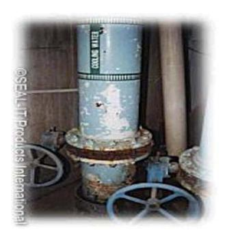
Fig. 3. Crevice Corrosion in a Flange
