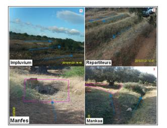
Fig. 1. Some illustrations of the components of the Meskat system
