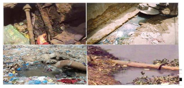
Figure.3.Drinking Water Pipes Passing Through Manholes/Drains
