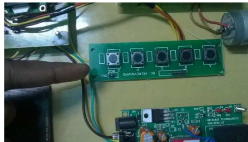
Fig 10 switch and motor
